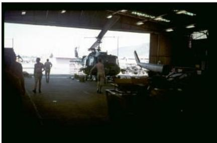
servicing aircraft and here is a main transmission being installed.
